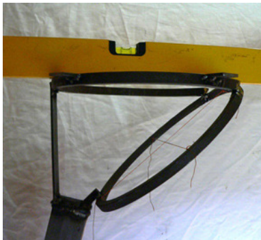
Fig. 67: C2 fixation with spirit level
