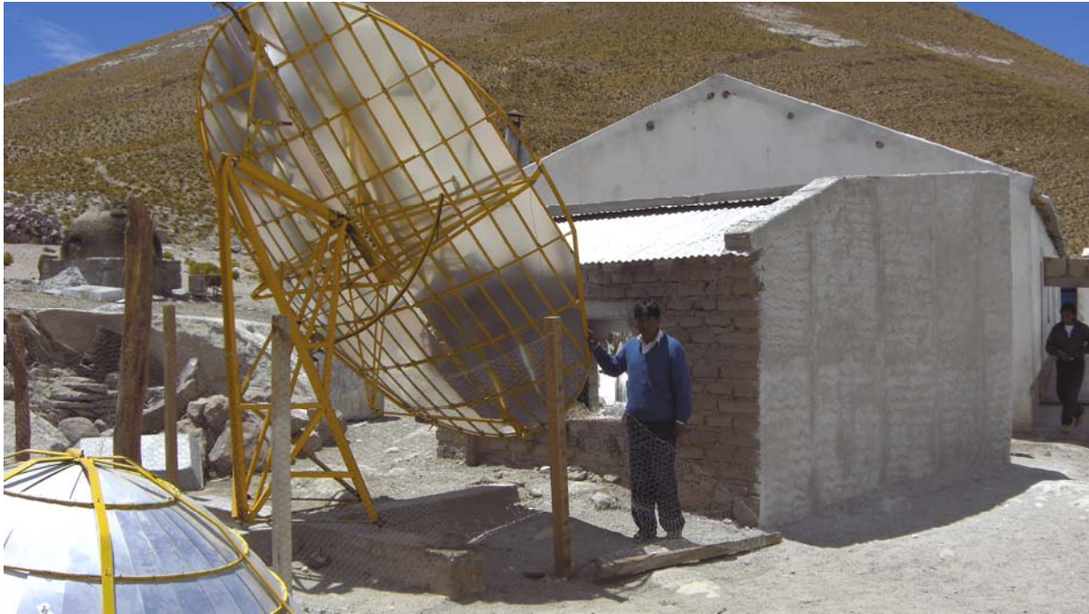
Fig.2: Solar community oven powered by Scheffler reflector
